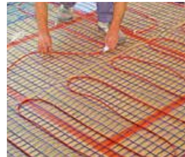
Heating cables connection.
