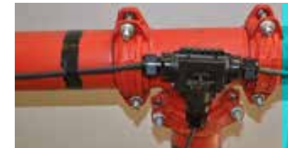
Connection of heating cables (Italy). Series TH211.
